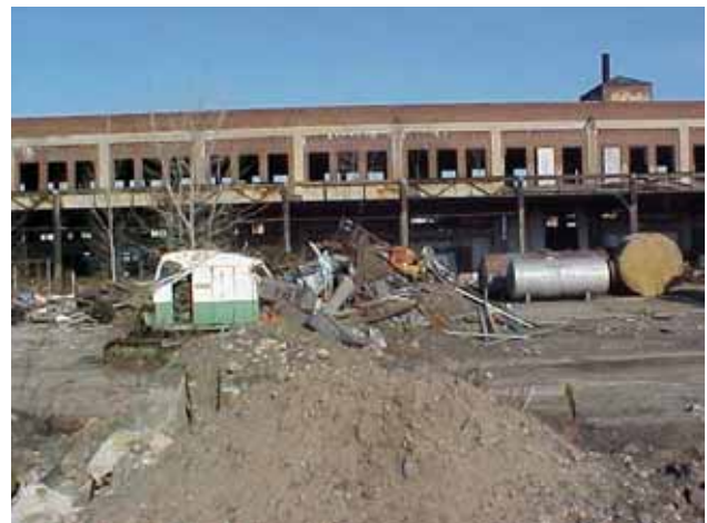
Pictured: REA Building at Sunnyside Yard prior to demolition.
