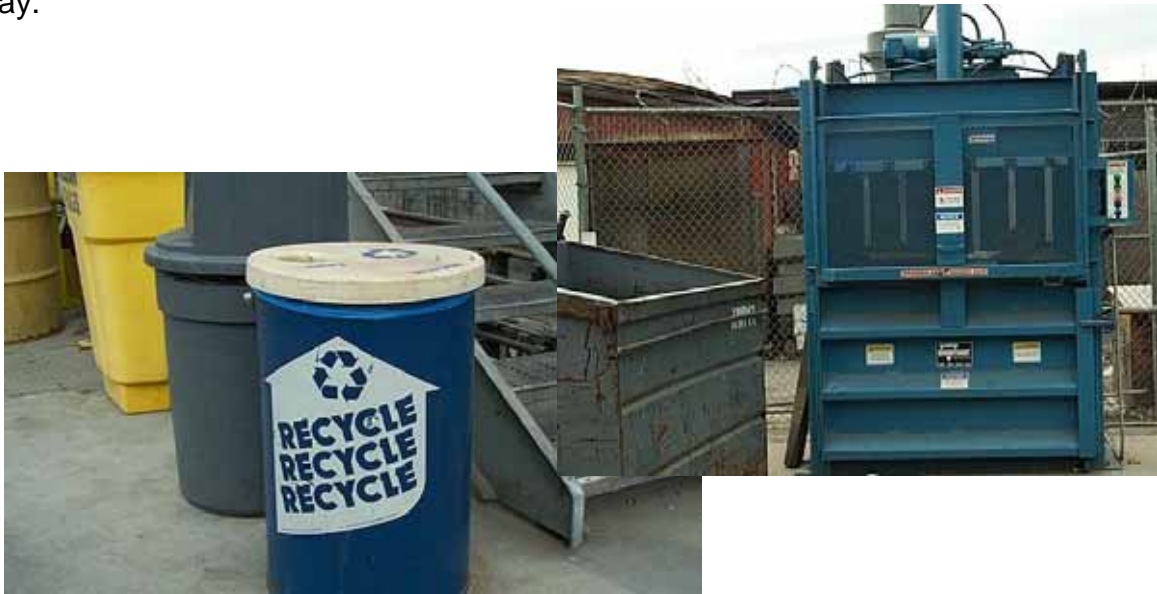
Pictured: Recycling bins and containers at Los Angeles Yard
